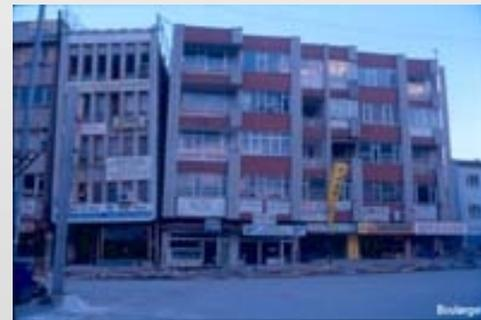
Tilt due to liquefaction (Adapazari)
